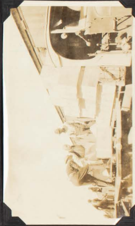
METHOD OF WORKING CASE OIL. TRAYS HOLDING 20-30 CASES ARE LIFTED FROM SHIP AND LANDED ON PLATFORM ALONGSIDE OF WHICH VEHICLE TO BE LOADED IS DRIVEN UP.
