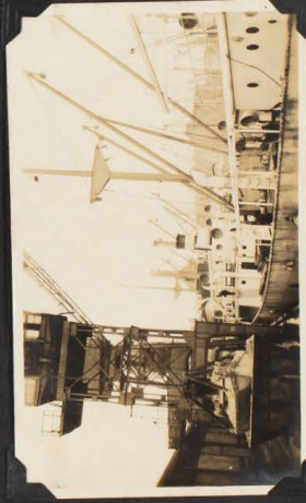
"M.V. BRAND" DISCHARGING BULK SULPHUR FROM GALVESTON, U.S.A., AT CENTRAL WHARF. RATE OF DISCHARGE, 40-50 TONS PER GRAB PER HOUR.
