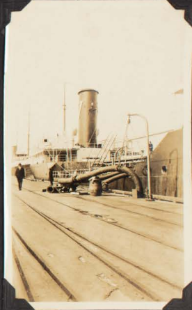
SS. PULPIT POINT DISCHARGING BULK MOTOR SPIRIT THROUGH A 10 INCH LEAD AT A RATE OF OVER 400 TONS PER HOUR.
