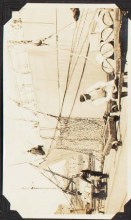
DISCHARGING SMALL PACKAGES OF MERCHANDISE ON WOODEN TRAYS IN ORDER TO AVOID DAMAGE BY CRUSHING AS WHEN SLUNG WITH ROPE.
