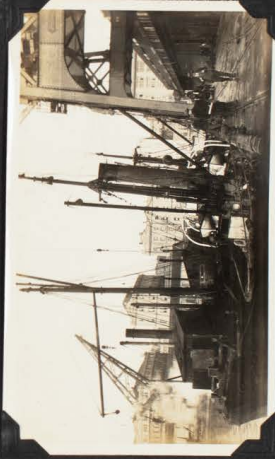
13 S.S. "WAIMEA" COALING FROM HULK ALONG- SIDE, BY MEANS OF CRANE & GRAB.
