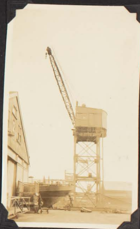
BABCOCK-WILCOX PORTAL CRANE. BOTH ABOVE CRANES LIFT UP TO 5 TONS AND HAVE A MAX. OUTRANGE FROM EDGE OF QUAY OF FEET.
