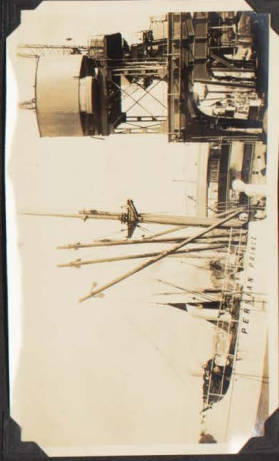
S.S. "PERSIAN PRINCE" DISCHARGING BULK ROCK PHOSPHATE FROM NAURU ISLAND AT KING'S WHARF. RATE OF DISCHARGE 30-40 TONS PER GRAB PER HOUR.
