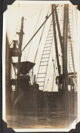
14 S.S. "KATANGATA" DISCHARGING COAL INTO HULK BY MEANS OF CRANE & GRAB WORK- ING INTO BIN, TRACK & TRAMLINE. AVERAGE 50 TONS PER HOUR APPROX.
