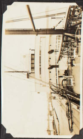
BRITISH IMPERIAL OIL COY'S METHOD OF DISCHARGING BY STEAM SUPPLIED TO SHIP'S PUMPS FROM BOILER HOUSE ASHORE. NOTE SMALLER HOSE CARRYING STEAM TO PUMPS. MOTOR SPIRIT DISCHARGED THROUGH 3 INCH LEADS AT 250-300 TONS PER HOUR.
