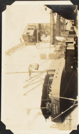
SS. ECHUNGA KING'S WHARF DISCHARGED 5,283 TONS OF NEWCASTLE COAL IN 3 DAYS 8 1/2 HRS. AVERAGE 1,428 TONS PER DAY FEBRUARY 1923.
