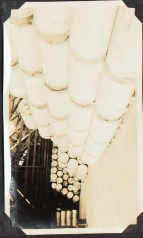
"NEWS PRINT", TOP FLOOR SHED 15, QUEEN'S WHARF. EACH REEL ABOUT 14 CWT, FLOOR LOAD 3 1/2 CWT PER FOOT.
