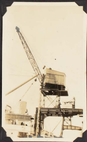
BABCOCK-WILCOX SEMI-PORTAL CRANE
