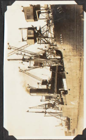
SS "KATOA" AS ABOVE, USING SEVEN CRANES AT FOUR SHIPS' GEARS; ELEVEN GANCS, RATE OF DISCHARGE 275 TONS PER HOUR, APPROX.
