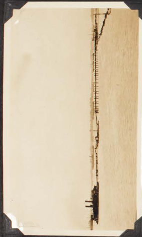
SUCTION DREDGER FILLING IN RECLAMATION ON WEST SIDE OF THE WESTERN WHARF FEB. 1929.
