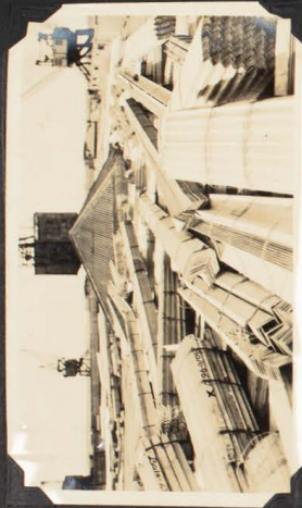
PART OF 600 TONS OF STEEL SECTIONS ON ROOF OF SHED 21 PRINCES WHARF FOR TRANSMISSION TOWERS, IN TRANSIT TO WAIKOKOPI, HAYNES BAY TO BE USED FOR CONVEYING CURRENT FROM WAIKAREMORUA HYDRO-ELECTRIC STATION.
