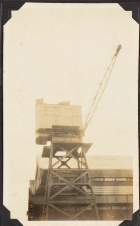
CARRICK "A" TYPE CRANE, MAX CAPACITY 5 TONS, OUTHANG
